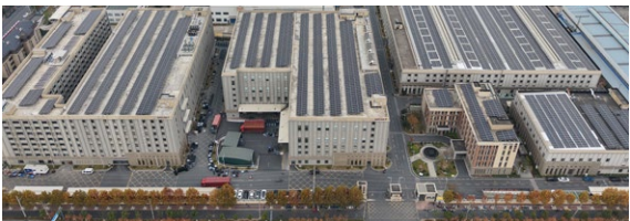
Rooftop solar PV system at the Hefei industrial park
